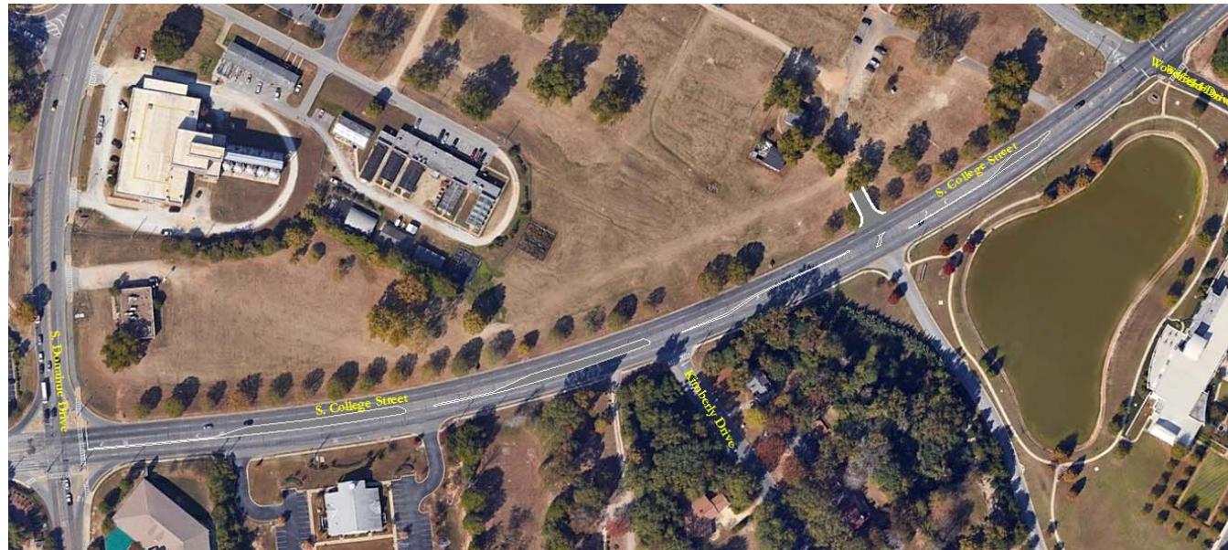
Figure 11 - S. College Street – S. Donahue Drive to Woodfield Drive Access – Existing Median Construction Project
